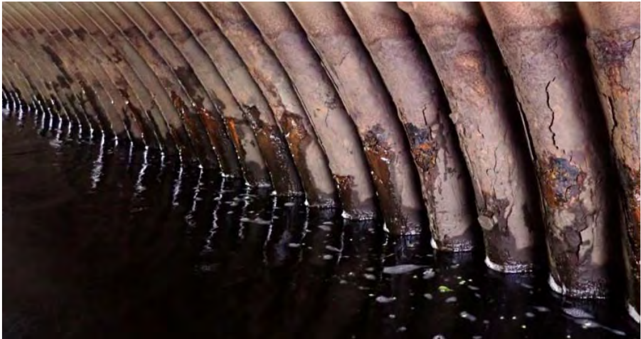
Figure 4: Area of Severe Deterioration in Span 1, Begin
