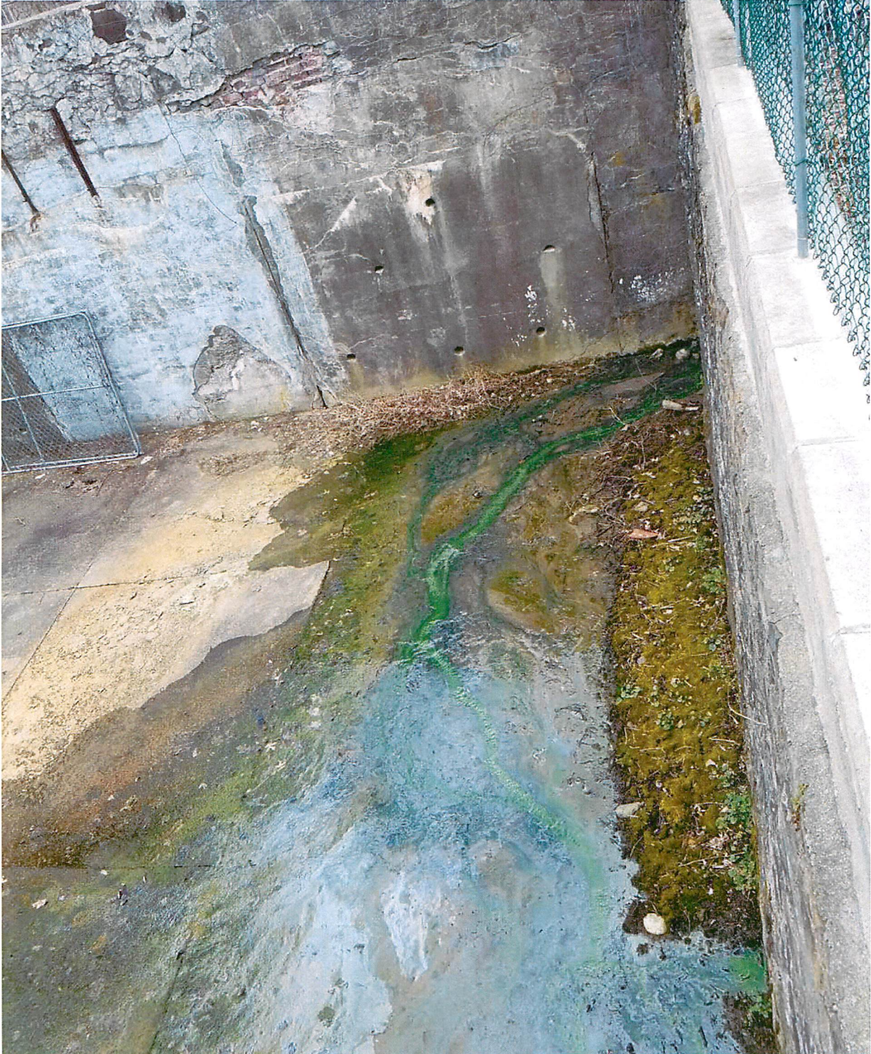
Attachment-1: Photo of sewage and dye discharging from retaining wall at 111 North Street
